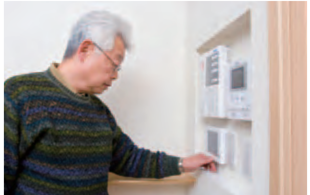
Checking the power generation monitor
