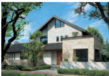
Is Stage Steel-frame detached house
