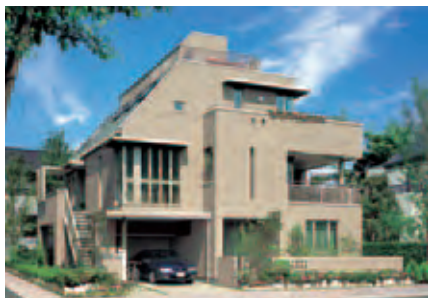
Biena Three-story Steel-frame house
